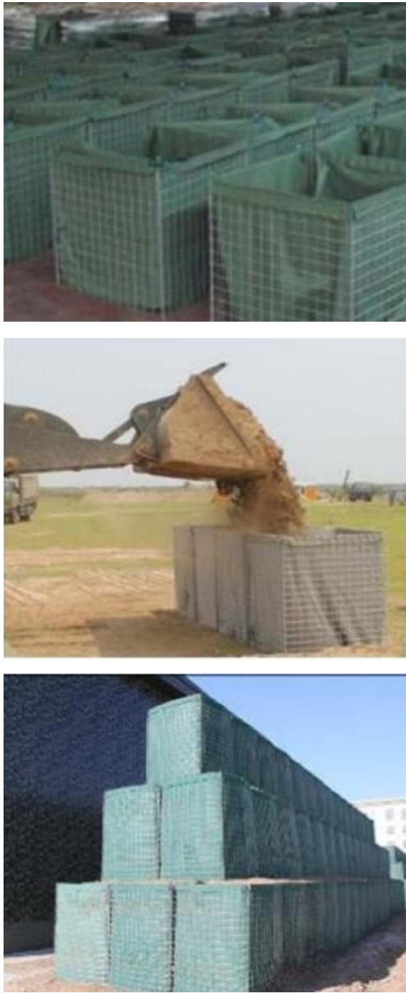
Figure 7. Rapid assembling anti-blast wall and Mechanical filling (Hongrui et al., 2021).
