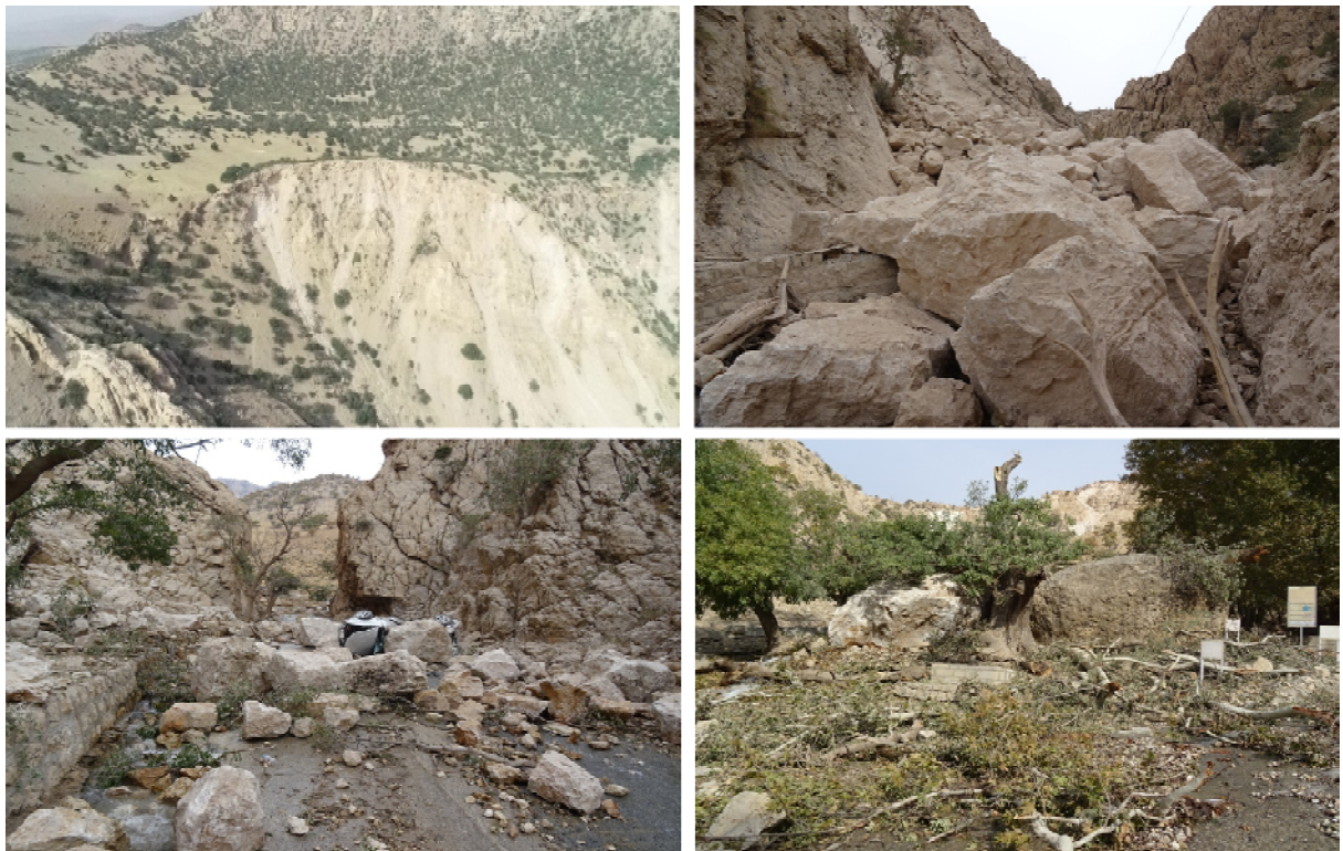
Figure 5. Images of Baba Yadegar rockfall zones.
