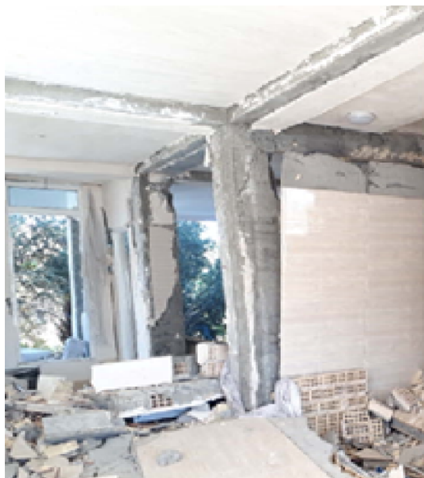
Figure 3. Lateral sway mechanism caused by formation of hinges on columns (Vetr et al., 2018).
