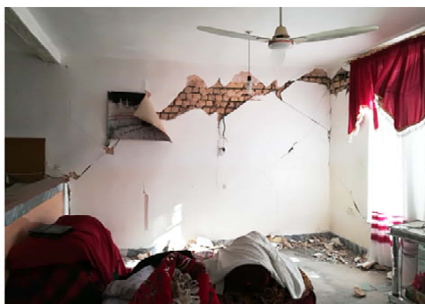
(b) Interior View of the Building
