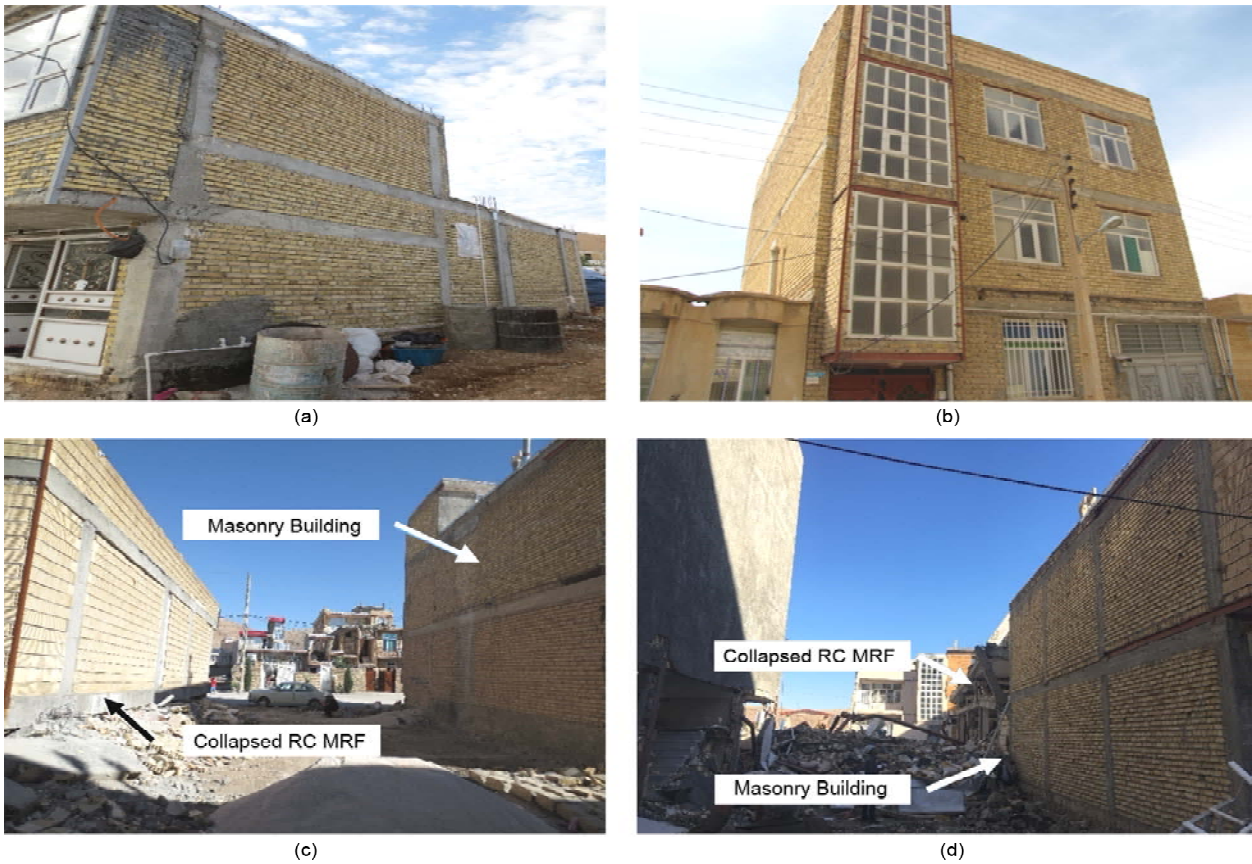
Figure 18. Instance of confined masonry buildings with good performance.
