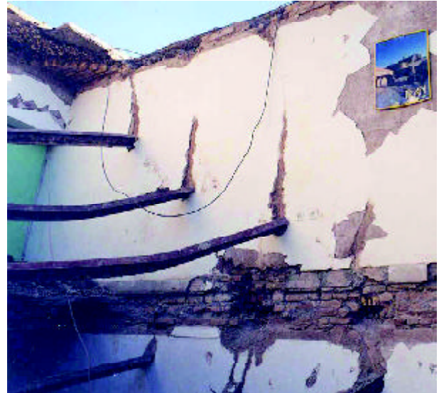
Figure 5. Collapse of jack arch steel beams as a result of small bearing length.
