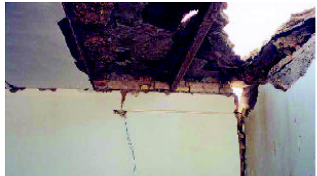
Figure 6. Collapse of masonry arches due to the movement of end support wall.
