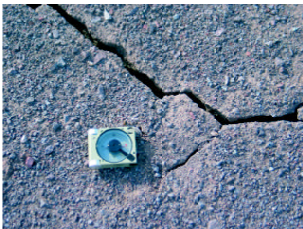
Figure 9. Tension cracks with 0.5 cm lateral displacement west of Baravat.
