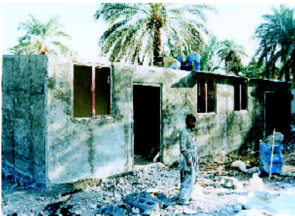
Figure 3. A sample of insitu-built temporary housing.
