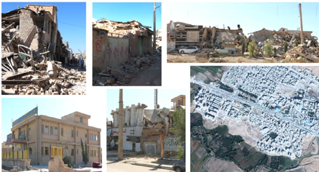
Figure 3. Damaged structures in Fooladi area.
