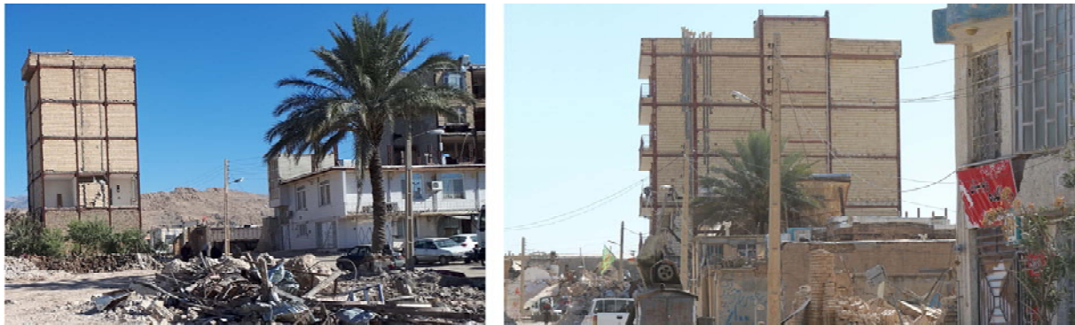
Figure 27. Buildings in eastern part of Fooladi area that survived the earthquake with minor damage.
