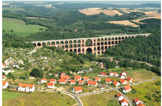
Figure 8. A view of Goltzschtal bridge.
