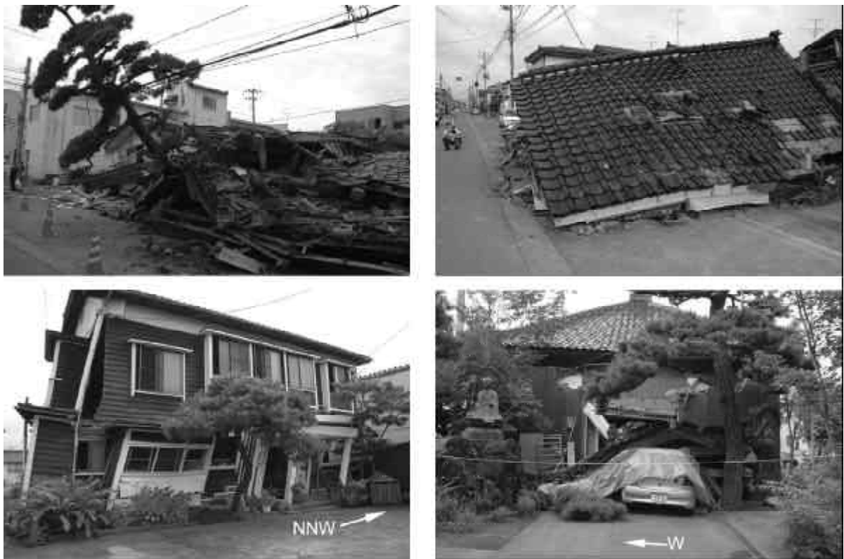
Figure 16. Observed damaged to the wooden houses in Highashi Hon Machi street together with their direction of collapsing.
