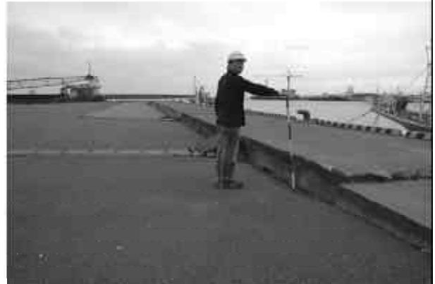
Figure 12. Damage to sheet pile type quay wall with tie rods in Kashiwazaki fishery port due to settlement where the evidence for liquefaction was also found.
