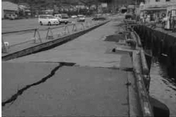
Figure 12. Damage to sheet pile type quay wall with tie rods in Kashiwazaki fishery port due to settlement where the evidence for liquefaction was also found.
