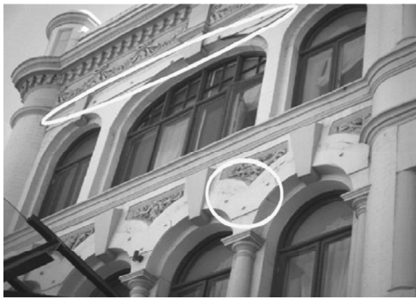
Figure 12. In-plane strengthening of masonry wall using bolted steel plates.
