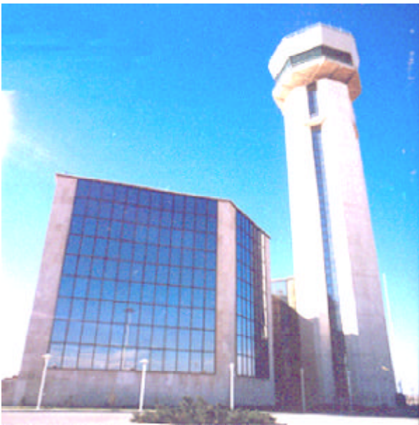
Figure 1. A typical control tower.
