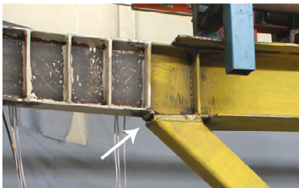
Figure 13. Brace to link connection fracture during Cycle 19.
