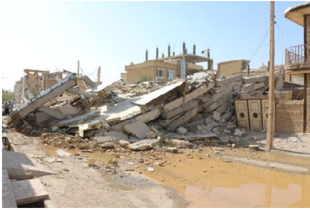
Figure 3. A pancake collapse in northern part of the study area due to the weakness of design and construction.
