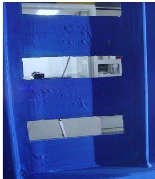
Figure 9. Yielding of infill plate at the back of shear panel in Sp-2 specimen at the 2% drift ratio.
