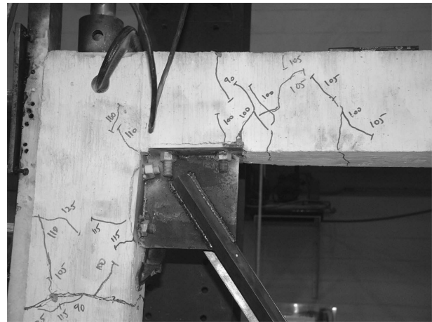
Figure 10. Photo of the braced frame, FX1, after the test.
