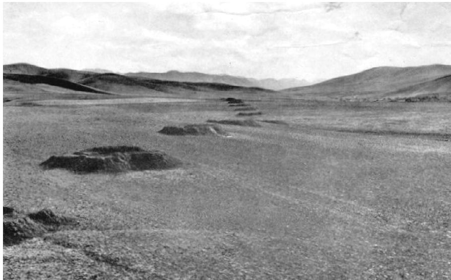
Figure 2. Example of a line of circular craters; Spoil from the excavation of the Qanat and from subsequent periods of maintenance is piled around the vertical access shafts to provide a wall to protect the shafts and the tunnel below from erosional damage from the inflow of water during a heavy desert rainstorm [1].
