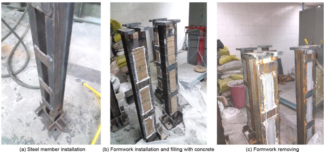
Figure 3. Construction process of concrete-filled specimens.
