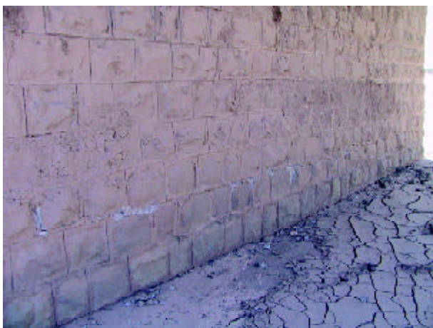
Figure 11. A bridge over the Posht-e-rud performed relatively well. There are signs of vertical movement in the base of the support walls/columns. Damage to pipelines is observed.
