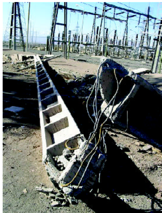
Figure 7. Damage to transmission line towers was not observed. Concrete and wooden poles are used to bring electricity from substations to users. Pole top transformers convert the electricity to 220V. Many distribution poles were damaged. A large number of distribution poles and street light poles were out of plumb after the earthquake.
