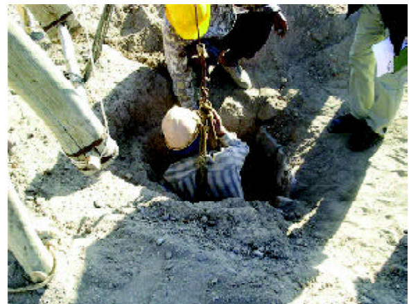
Figure 6. The vertical wells, also used as access wells, are usually large enough for one person to be able to climb down (about 90cm across). Note the use of old tire at the entrance of one well. Damage to the qanat systems included underground tunnel collapse and closure (not shown), access well failure, which in turn causes the closure of the underground tunnel, damage to the channels. At the time of our visit a number of qanat builders had been brought from other parts of country to repair the very important qanats.
