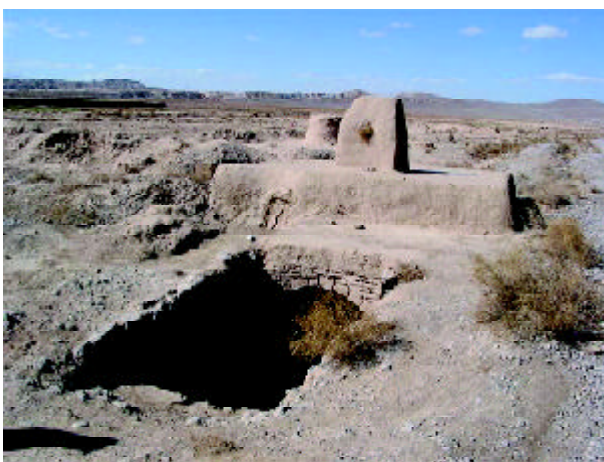
Figure 5. Once the qanat chain arrives at its destination, the underground tunnel reaches the ground surface (top and middle left pictures). From there the water is distributed via man-made channels and brought to farms and date palm gardens. Damage to the channels is noted in the middle and lower right pictures. The qanat water sometime is stored in traditional underground reservoirs (bottom two pictures).
