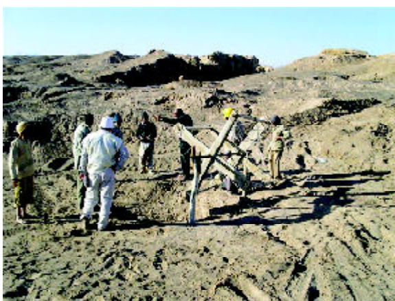
Figure 6. The vertical wells, also used as access wells, are usually large enough for one person to be able to climb down (about 90cm across). Note the use of old tire at the entrance of one well. Damage to the qanat systems included underground tunnel collapse and closure (not shown), access well failure, which in turn causes the closure of the underground tunnel, damage to the channels. At the time of our visit a number of qanat builders had been brought from other parts of country to repair the very important qanats.
