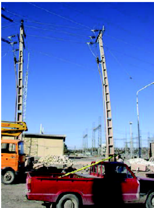
Figure 7. Damage to transmission line towers was not observed. Concrete and wooden poles are used to bring electricity from substations to users. Pole top transformers convert the electricity to 220V. Many distribution poles were damaged. A large number of distribution poles and street light poles were out of plumb after the earthquake.
