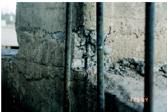
Figure 1. Elevated concrete water tank located in near the old section of the city where the damage was high. The tank experienced severe stress and deformation at the column-beam connections.
