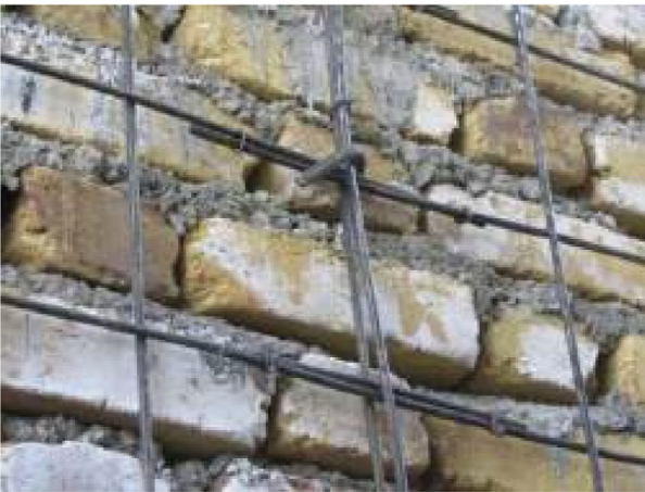
(c) U-shaped Shear Dowel Bars
