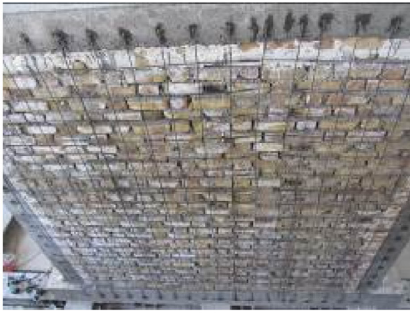
(a) Fixing the Steel Mesh into the Drilled Holes
