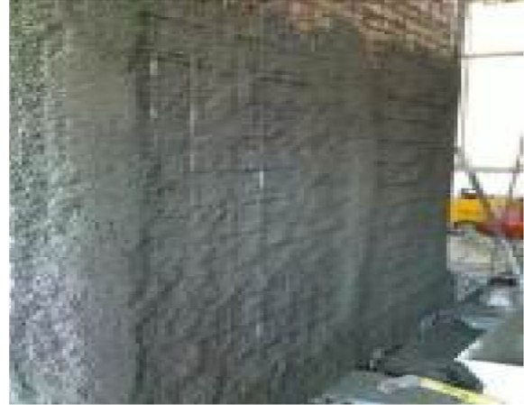
(b) Concreting the Wall
