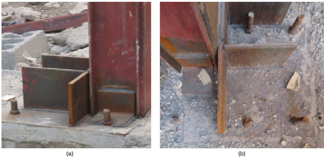
Figure 17. Common base plate construction practice in earthquake affected areas.
