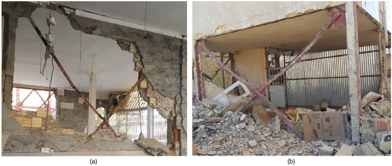
Figure 6. Overall buckling of slender brace members.
